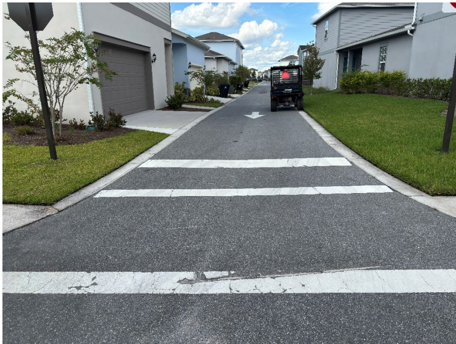
Photo 30 - Marconi Alley – Deterioration of Thermoplastic and Gouged Asphalt
