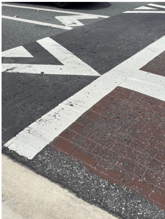
Photos 16 & 17 - Deteriorating Thermoplastic and Worn Coloration
