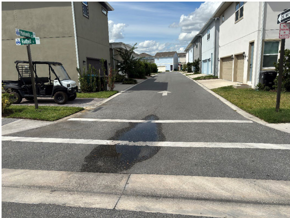
Photo 23 - Markowitz Alley – Ponding Water
