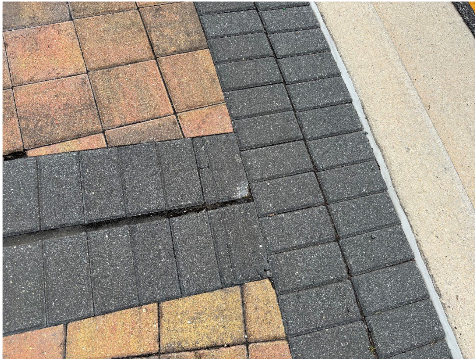
Photo 9 - Chipped Concrete Pavers on Truck Apron
