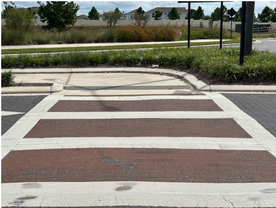
Photo 19 - Deteriorating Thermoplastic and Worn Coloration
