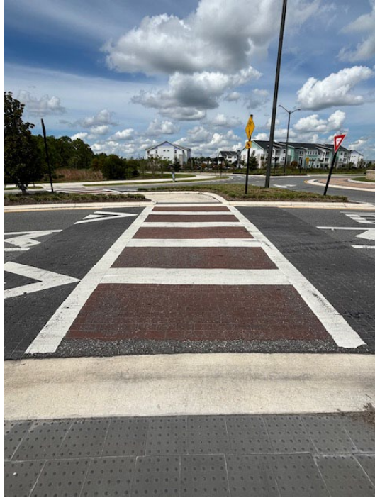
Photos 14 & 15 - Deteriorating Thermoplastic and Worn Coloration
