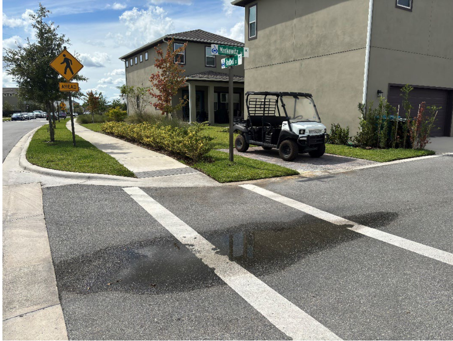
Photo 22 - Markowitz Alley – Ponding Water
