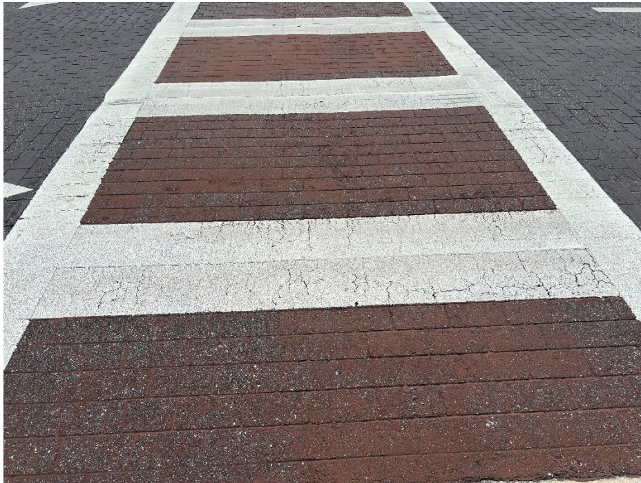
Photo 11 - Deteriorating Thermoplastic and Worn Coloration
