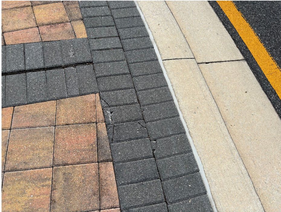
Photo 8 - Broken Concrete Pavers on Truck Apron
