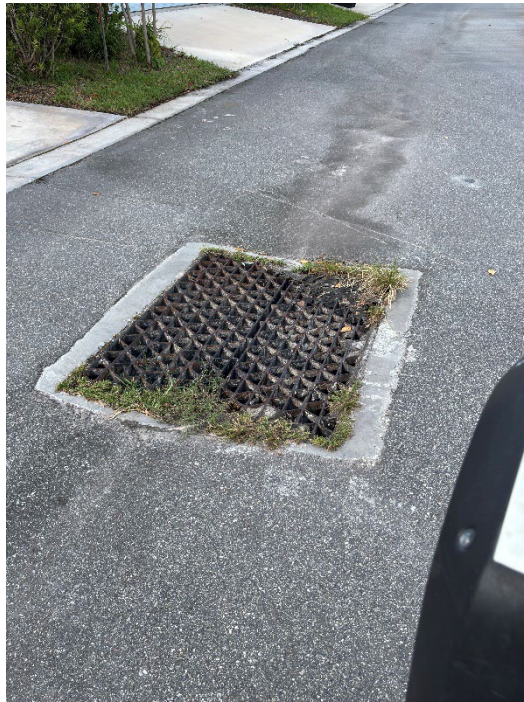
Photo 31 - Bragg Alley – Overgrowth on Inlet Top
