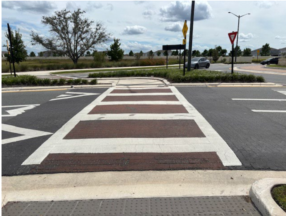
Photo 20 - Deteriorating Thermoplastic and Worn Coloration
