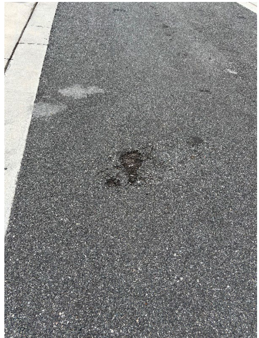
Photos 24 & 25 - Laggett Alley – Asphalt Damage
