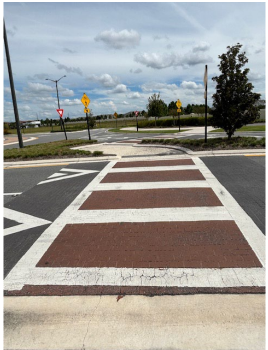
Photos 16 & 17 - Deteriorating Thermoplastic and Worn Coloration
