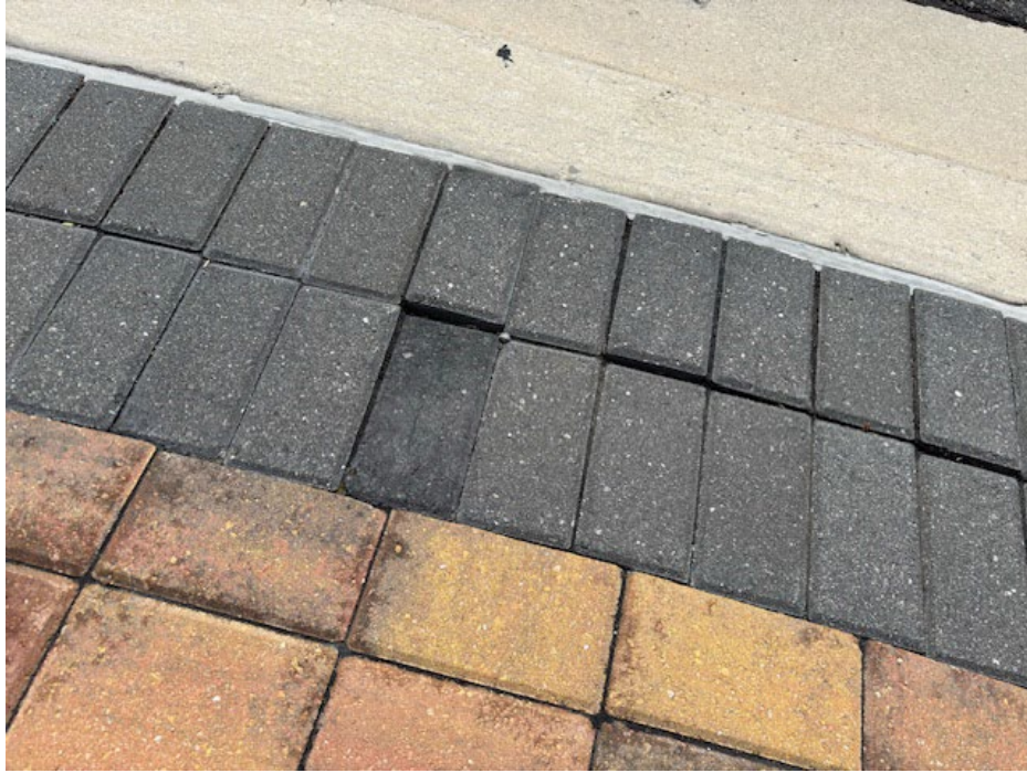
Photo 18 - Uneven Concrete Pavers on Truck Apron
