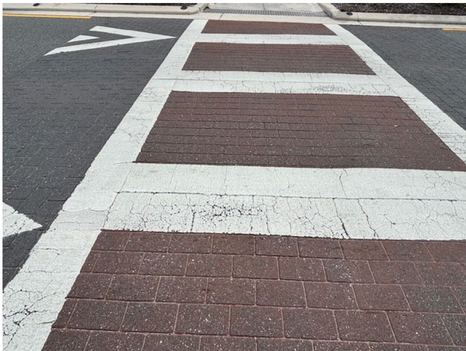
Photo 5 - Deteriorating Thermoplastic and Worn Coloration
