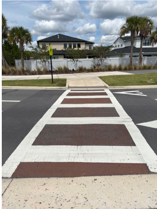
Photo 10 - Deteriorating Thermoplastic and Worn Coloration
