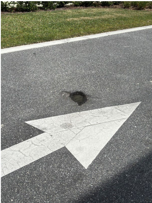
Photos 26 & 27 - Laggett Alley – Asphalt Damage
