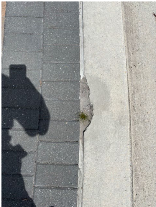
Photos 2 & 3 - Damage to the Concrete Curb Along Truck Apron
