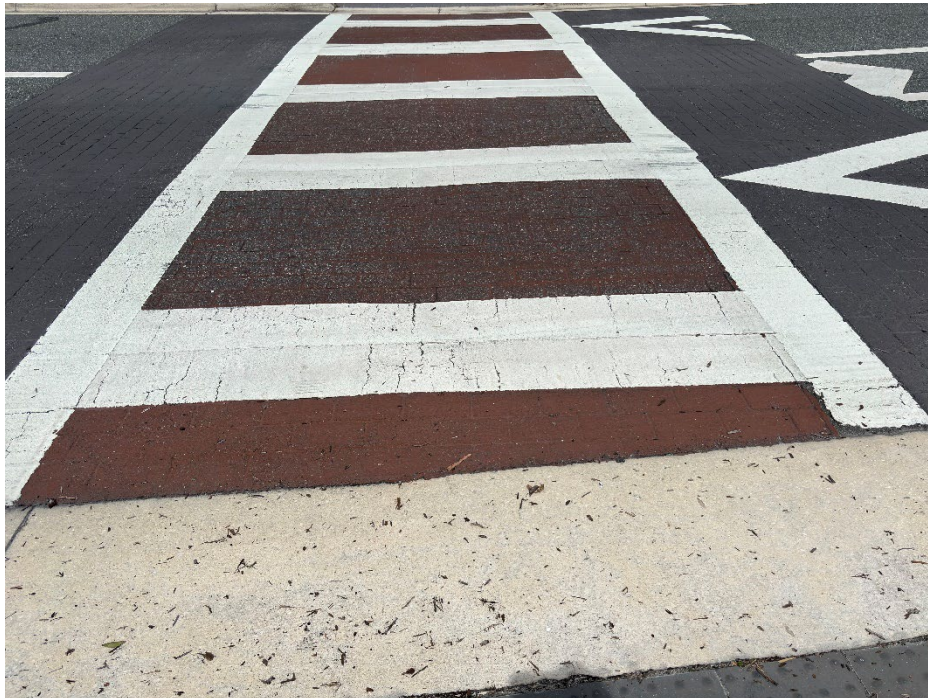
Photos 13 - Deteriorating Thermoplastic and Worn Coloration
