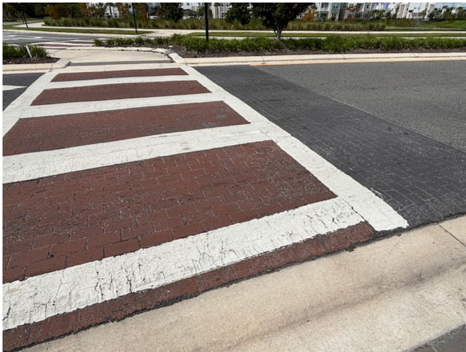
Photo 21 - Deteriorating Thermoplastic and Worn Coloration
