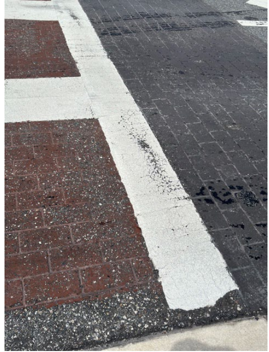
Photos 14 & 15 - Deteriorating Thermoplastic and Worn Coloration
