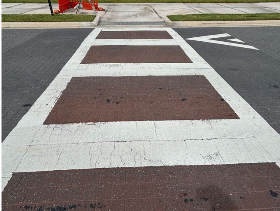
Photo 4 – Deterioration of Thermoplastic and Worn Coloration
