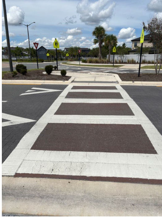
Photo 12 - Deteriorating Thermoplastic and Worn Coloration
