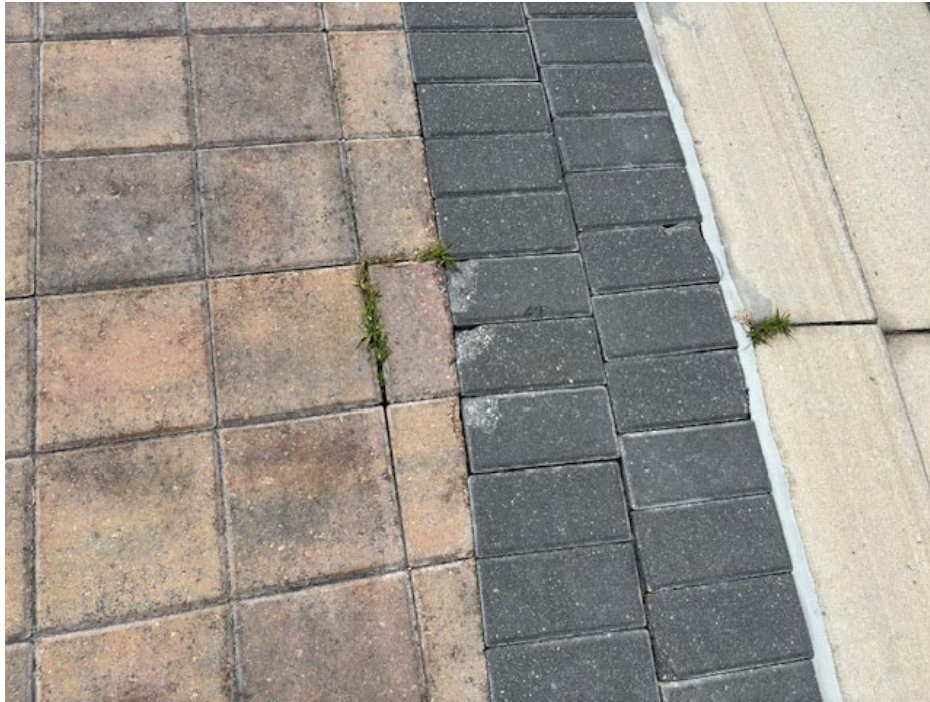
Photo 6 - Chipped Concrete Pavers on Truck Apron
