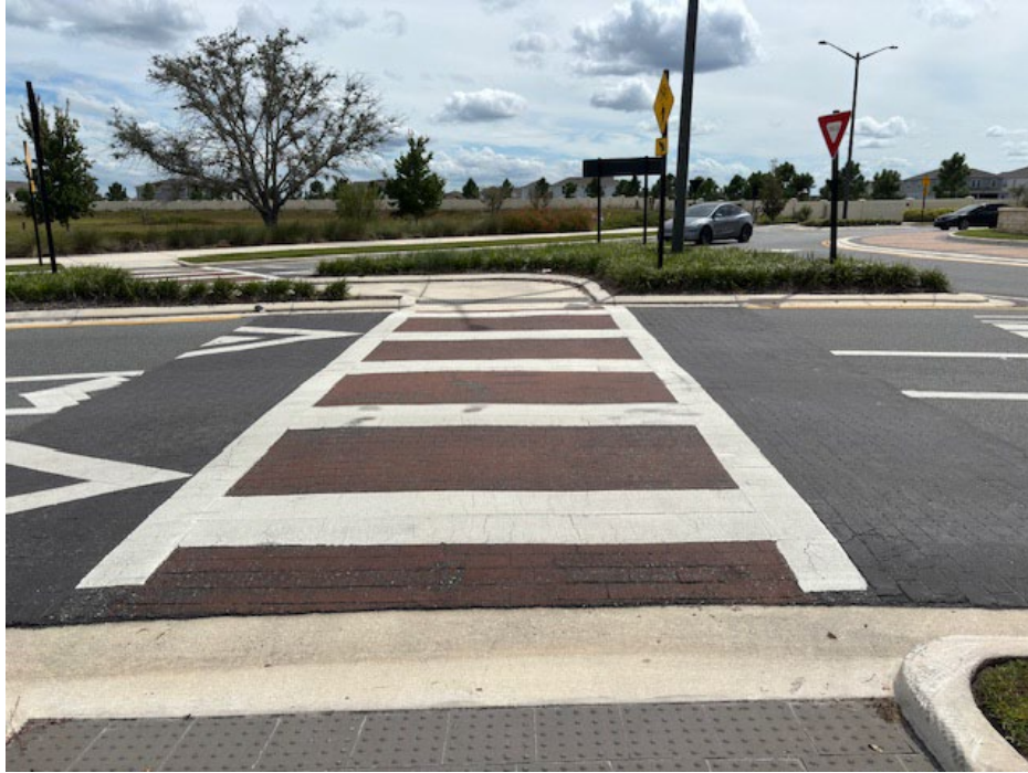
Photo 20 - Deteriorating Thermoplastic and Worn Coloration
