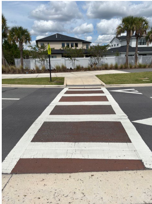
Photo 10 - Deteriorating Thermoplastic and Worn Coloration
