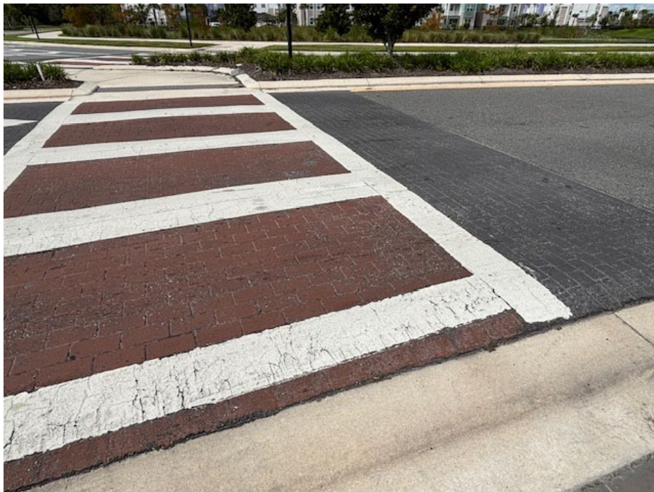
Photo 21 - Deteriorating Thermoplastic and Worn Coloration
