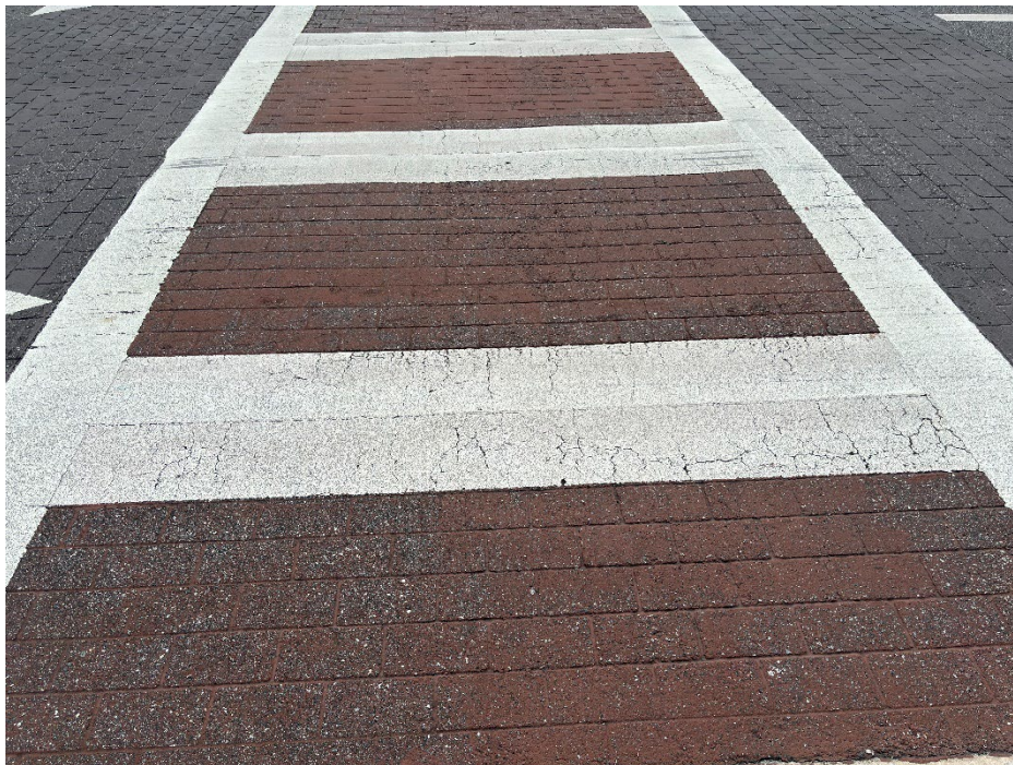
Photo 11 - Deteriorating Thermoplastic and Worn Coloration
