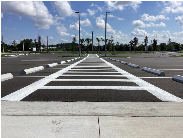
Recently Completed Work (4)
