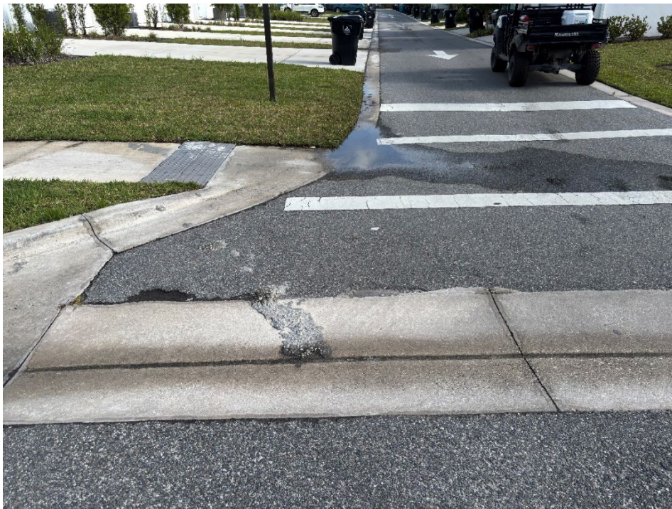
Photo 16.1 - Bragg Alley – Low Spot in Ribbon Curb, Concrete on Valley Gutter (New Photo – 2026 Assessment)
