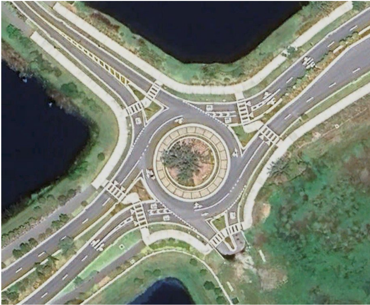
AERIAL PHOTO Roundabout at Luminary Boulevard and Selten Way
