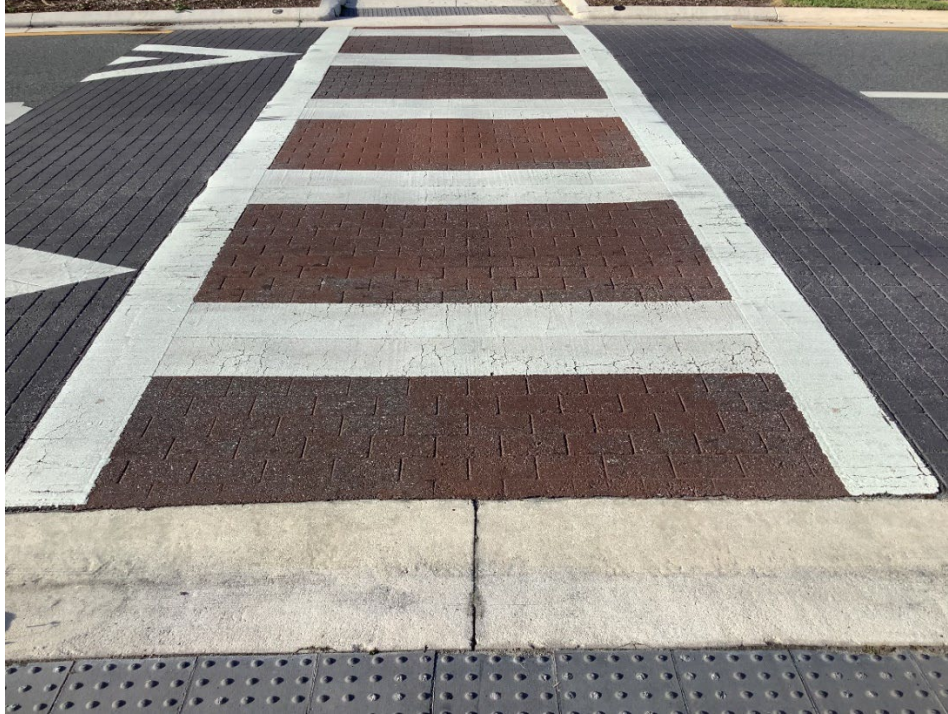
Photo 6 - Deteriorating Thermoplastic and Worn Coloration (No Observed Changes) (Refer to Prior Photo 11 – 2025 Assessment)
