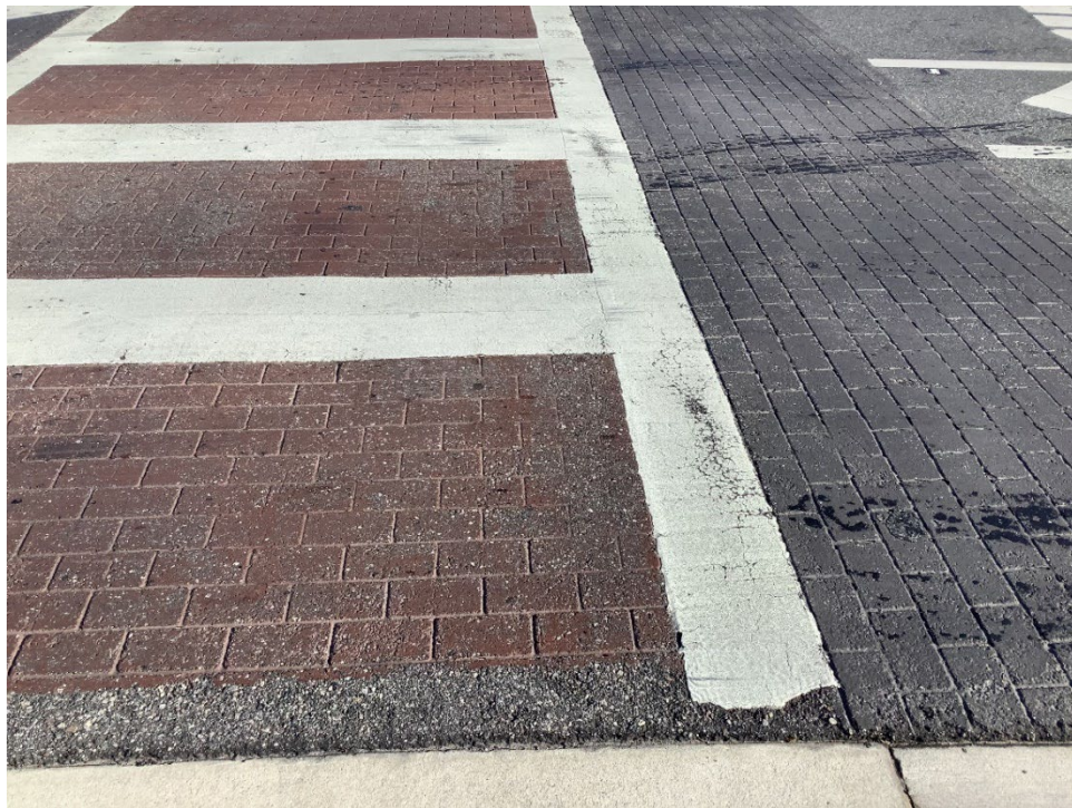
Photo 9 - Deteriorating Thermoplastic and Worn Coloration (No Observed Changes) (Refer to Prior Photo 15 – 2025 Assessment)
