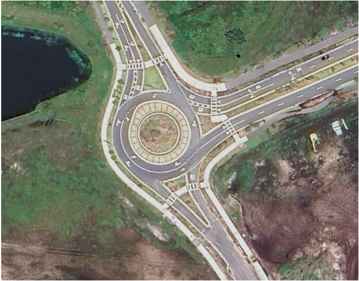
AERIAL PHOTO Roundabout at Centerline Drive and Luminary Boulevard
