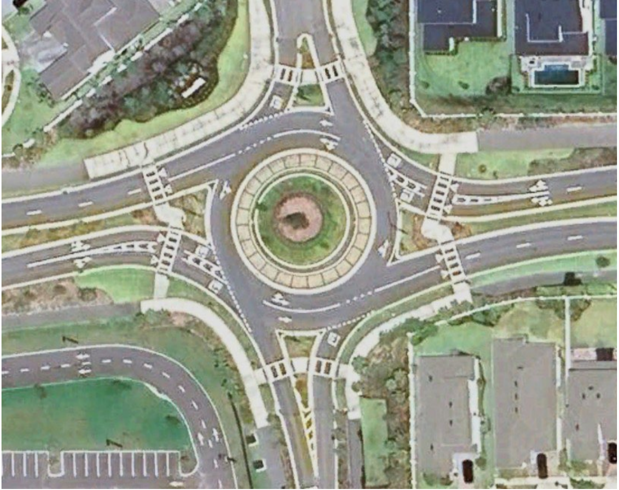
AERIAL PHOTO Roundabout at Luminary Boulevard and Pearson Avenue
