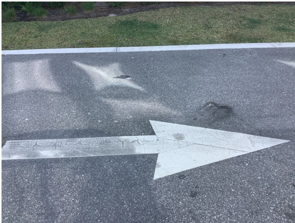
Photo 13- Laggett Alley – Asphalt Damage (No Observed Changes) (Refer to Prior Photo 27 – 2025 Assessment)
