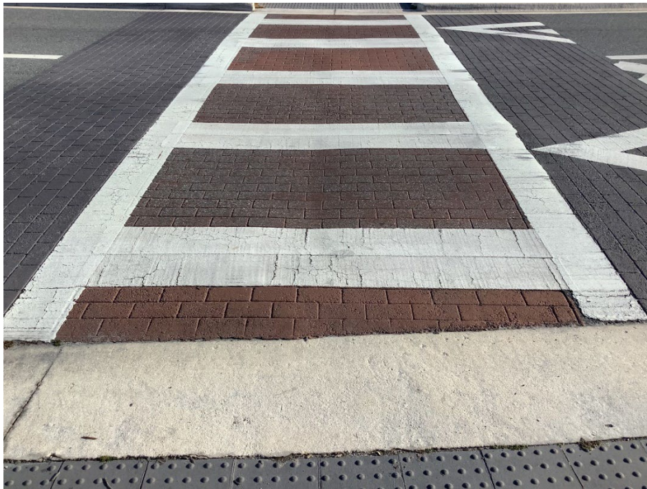
Photo 7 Deteriorating Thermoplastic and Worn Coloration (Further Deterioration Observed) (Refer to Prior Photo 13 – 2025 Assessment)
