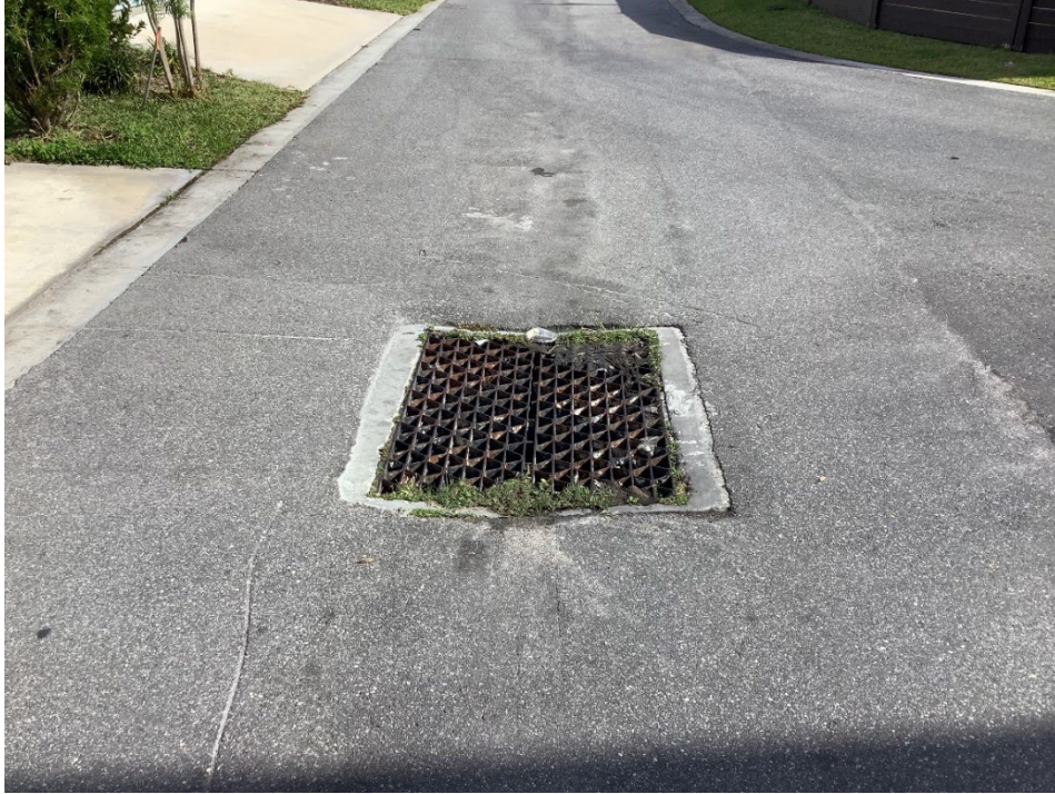
Photo 16 - Bragg Alley – Scarred Asphalt (No Observed Changes) (Refer to Prior Photo 31 – 2025 Assessment)
