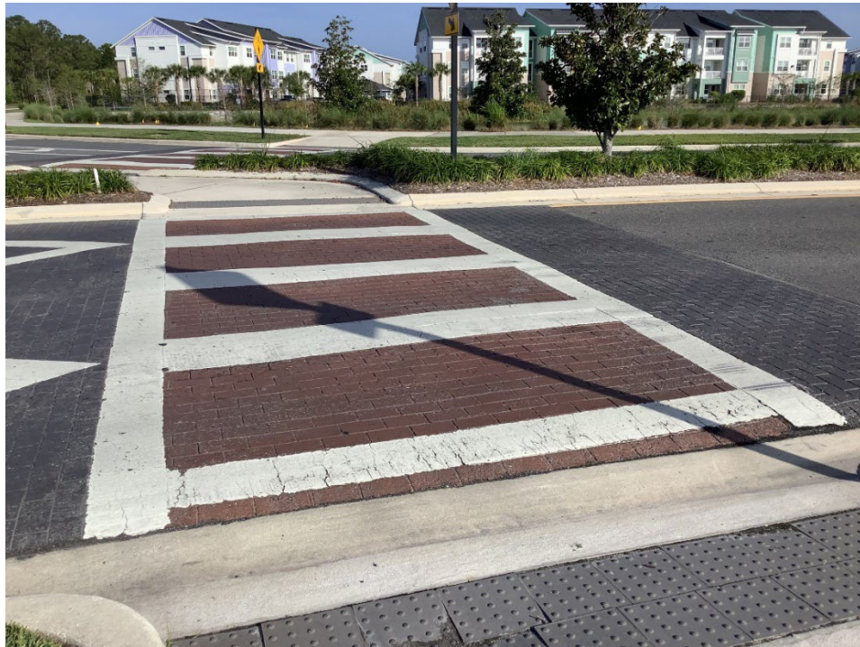
Photo 11 Deteriorating Thermoplastic and Worn Coloration (Further Deterioration Observed) (Refer to Prior Photo 21 – 2025 Assessment)
