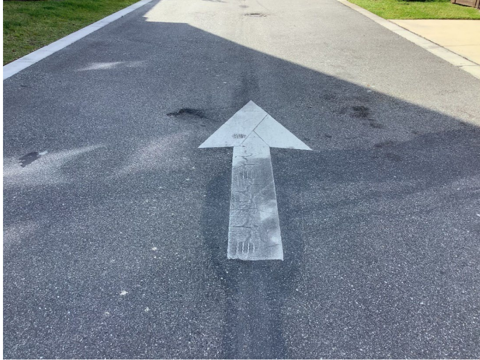
Photo 12 - Laggett Alley – Asphalt Damage (No Observed Changes) (Refer to Prior Photo 26 – 2025 Assessment)
