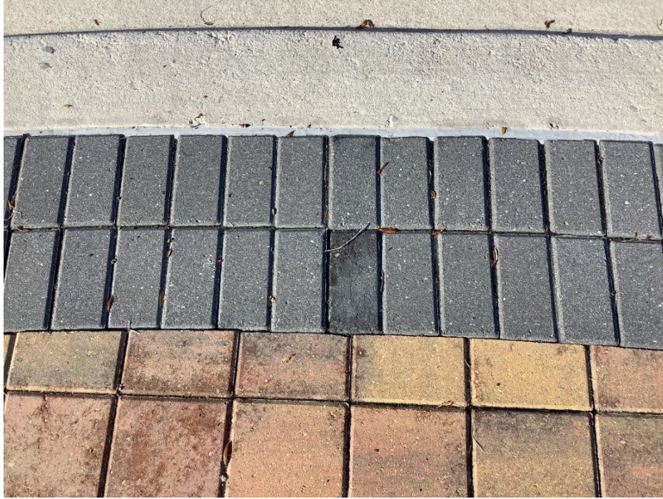
Photo 10 - Uneven Concrete Pavers on Truck Apron (No Observed Changes) (Refer to Prior Photo 18 – 2025 Assessment)
