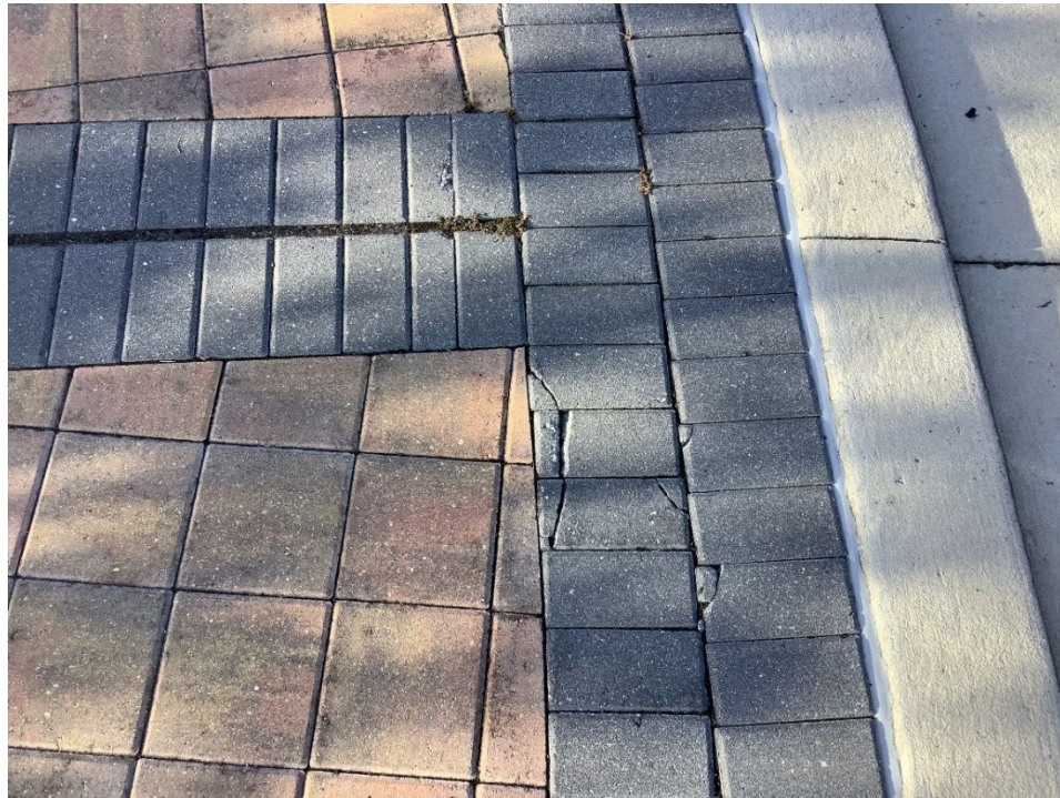
Photo 5 - Broken Concrete Pavers on Truck Apron (Increased Damage Observed) (Refer to Prior Photo 8 – 2025 Assessment)
