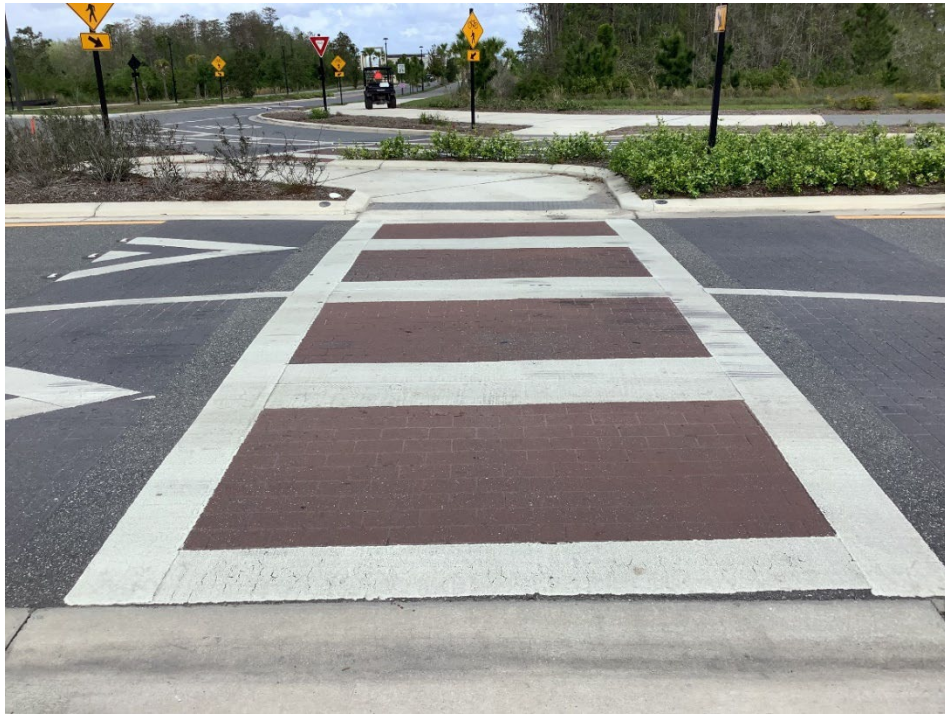
Photo 3 - Deterioration of Thermoplastic and Worn Coloration (No Observed Changes) (Refer to Prior Photo 5 – 2025 Assessment)
